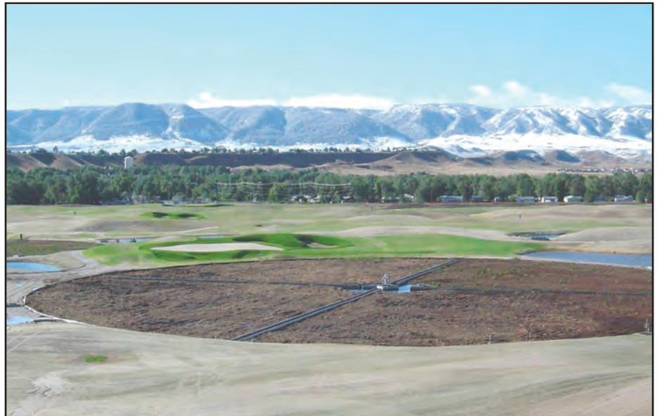
**This radial-flow wetland cell at Casper, Wyoming is insulated and aerated for year-round operation at temperatures as low as -35°F. (Photo courtesy of the RETEC Group, Inc.)**
