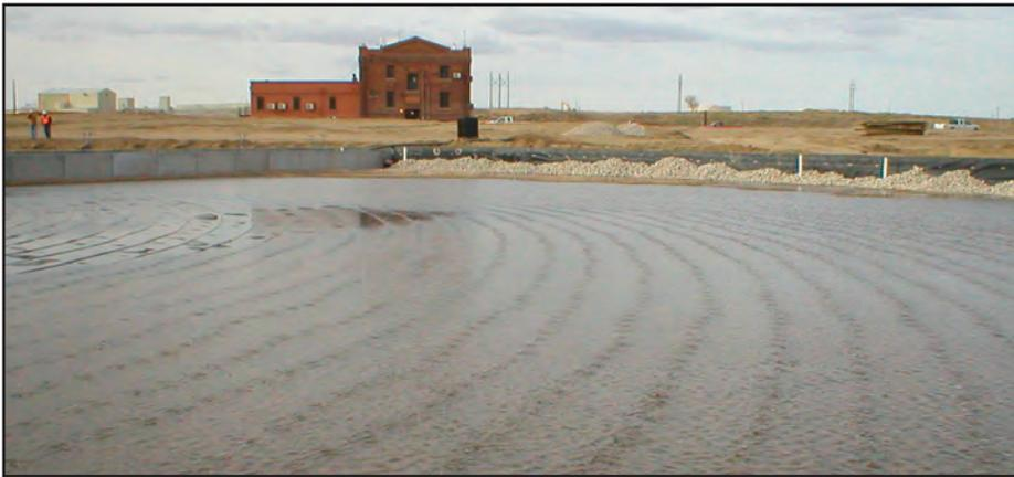
**The Casper wetlands use a patented aeration process (Forced Bed Aeration™) to achieve extremely uniform air distribution in the wetland cells.**
