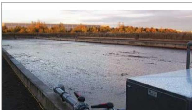
Full scale demonstration of wetland aeration for treatment of deicing fluid from Heathrow Airport in London
